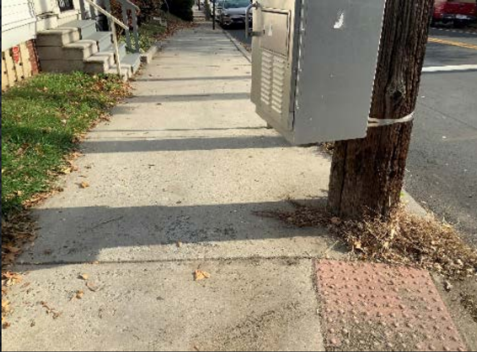
EXISTING OBSTRUCTION - SCOPING
